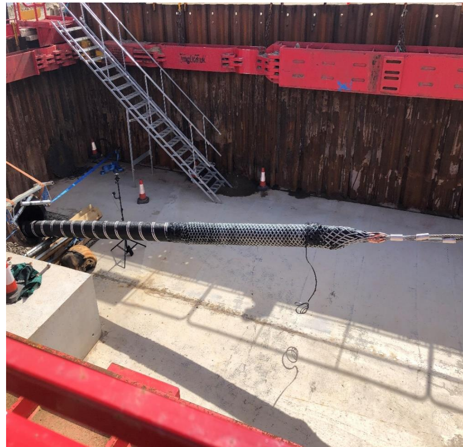
Offshore export cable pull at landfall
