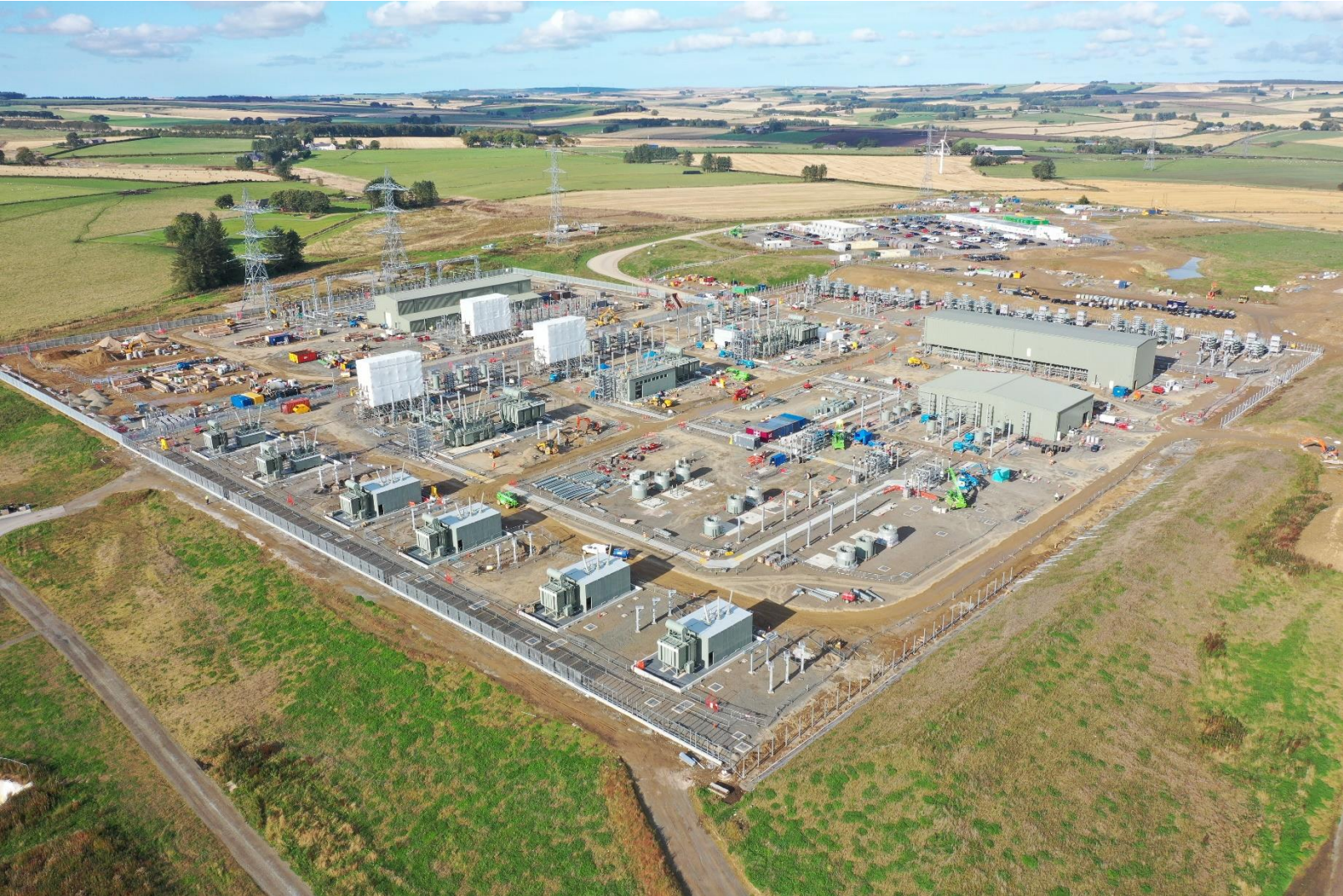
Onshore substation aerial view
